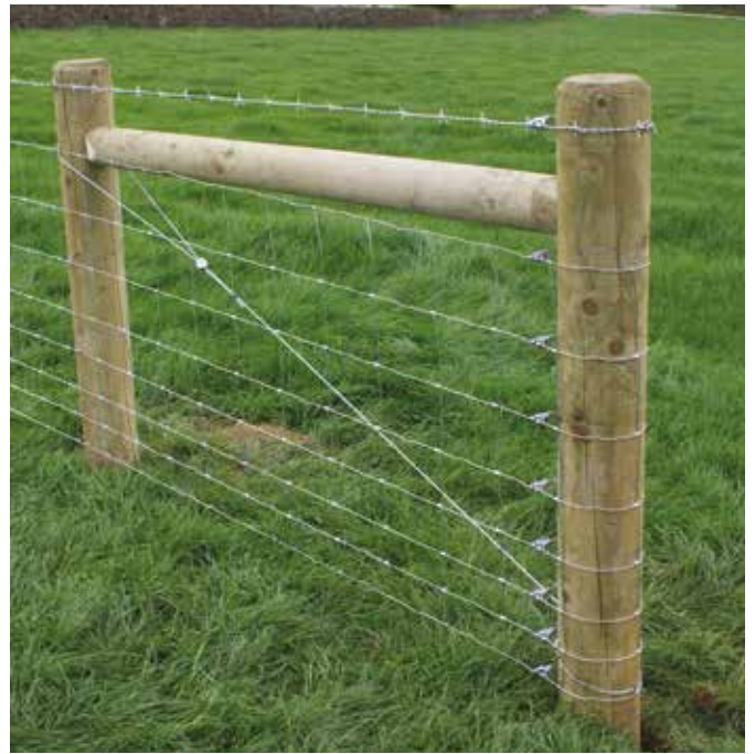
FPAK - Installed on a H end post
